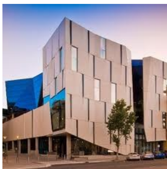
Hawke Building, University of South Australia City West Campus
